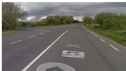
Fig 2: Google Maps image of the N53 near Rassan
